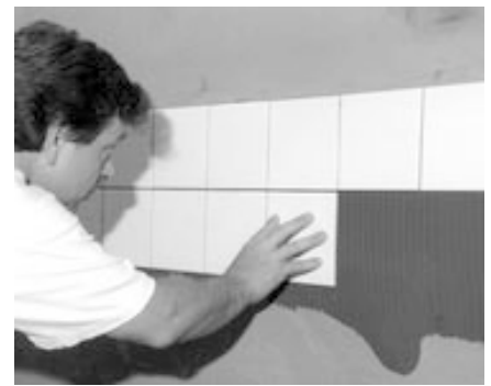
Figure 8. Application of a thin-bed ceramic tile adhesive (spreading the adhesive mortar with a notched trowel on a wall to be covered with ceramic tiles); picture: Wacker Polymer Systems
